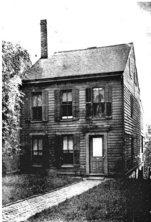
Scriber House needing paint
