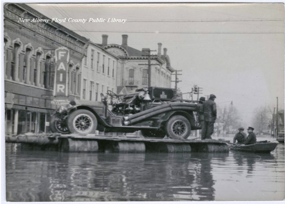
A firetruck on oil drums on East Market Street
