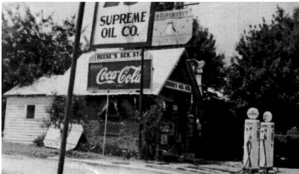
Early service station on U.S. 150
