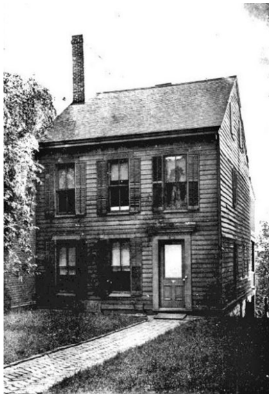
Scribner House needing paint
