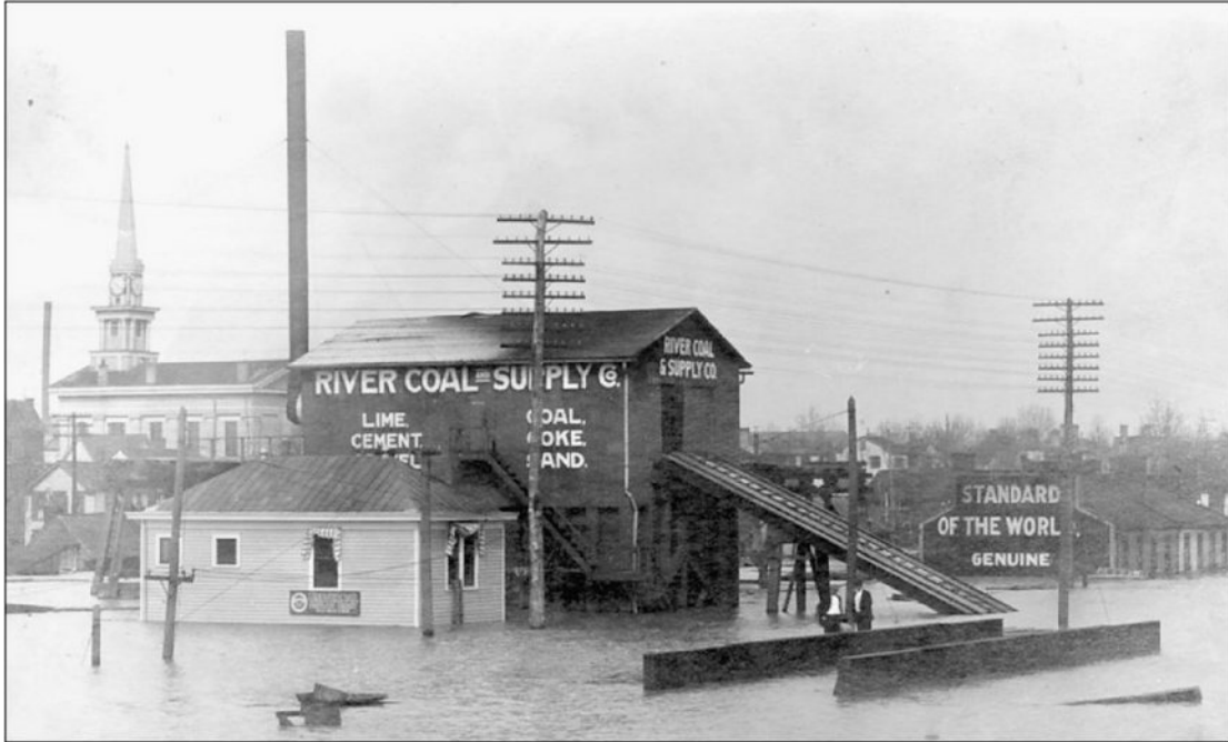
Note the Town Clock Church has its original steeple
